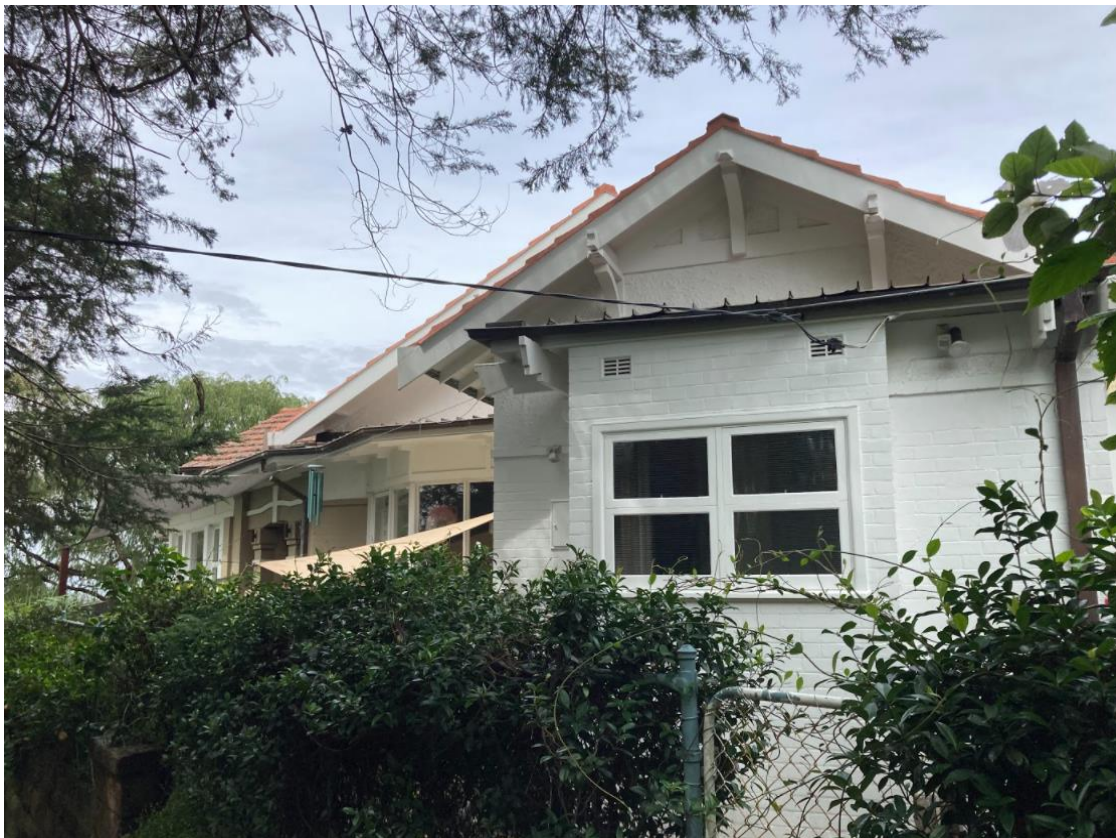
Figure 6: 27 Riddell Street, viewed from raised pedestrian pathway.
