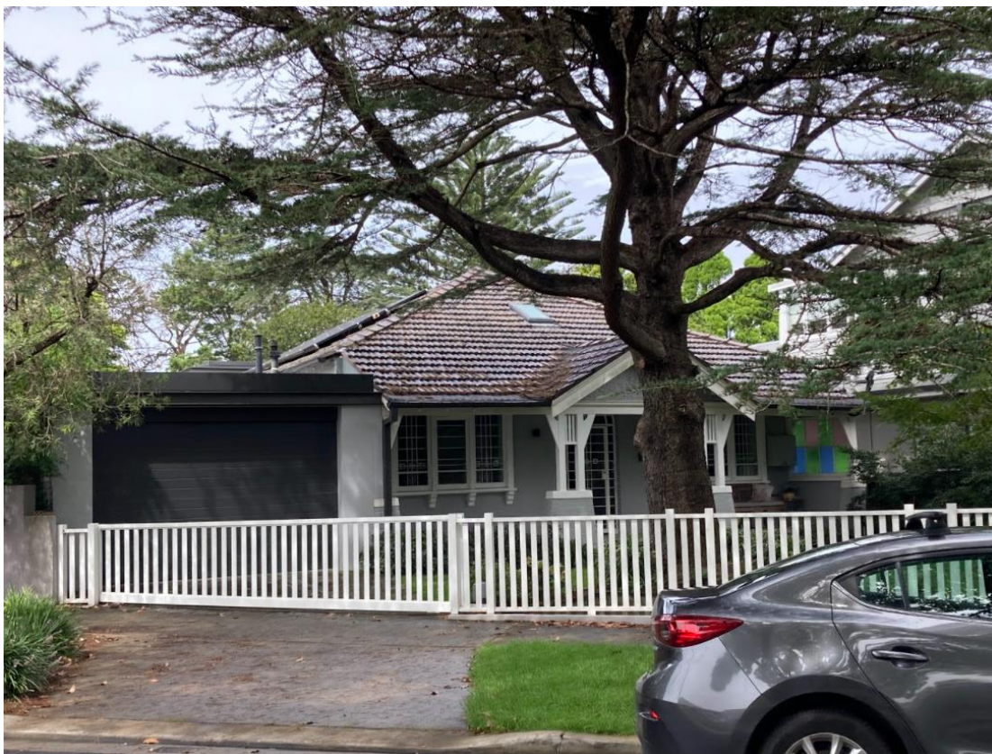
Figure 4: 15 Riddell Street, viewed from street frontage.
