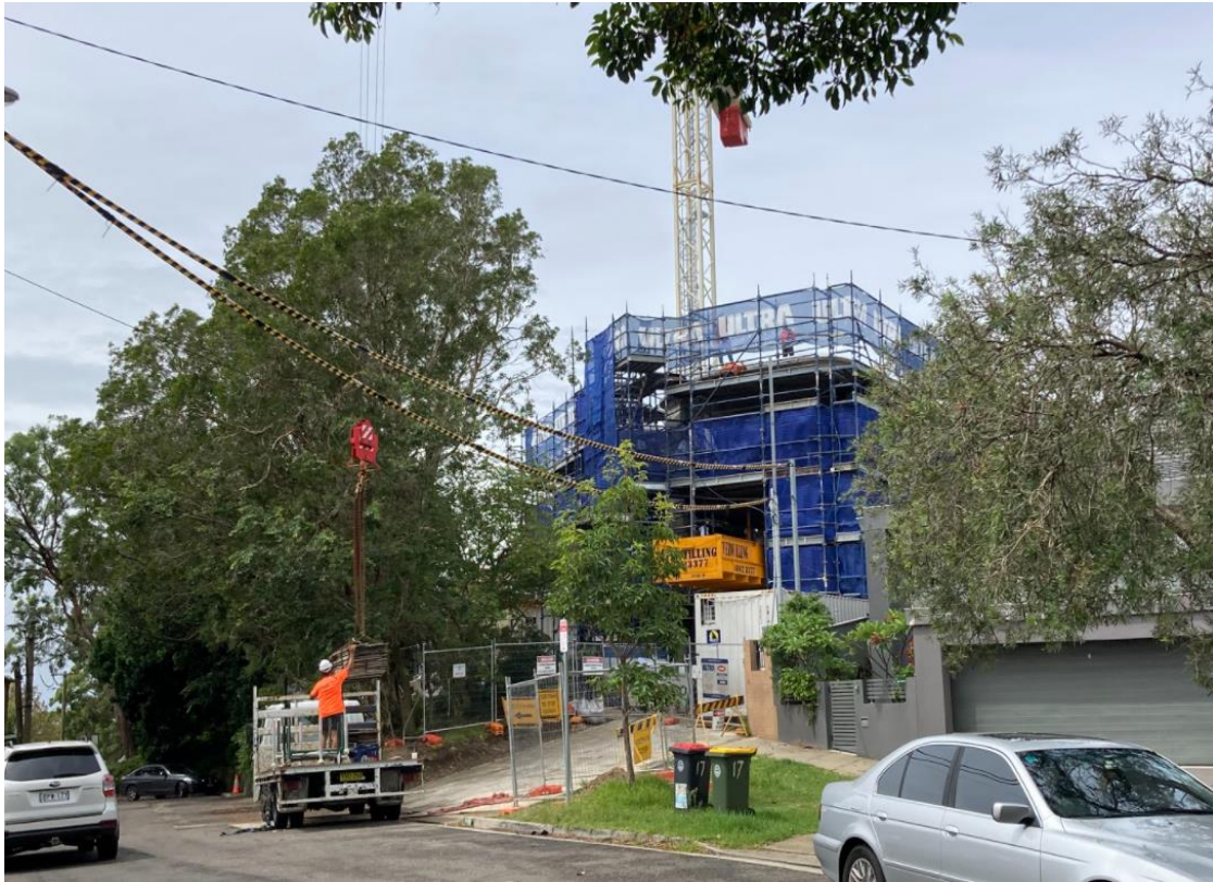
Figure 5: Apartments under construction at 21-23 Riddell Street, viewed from street.
