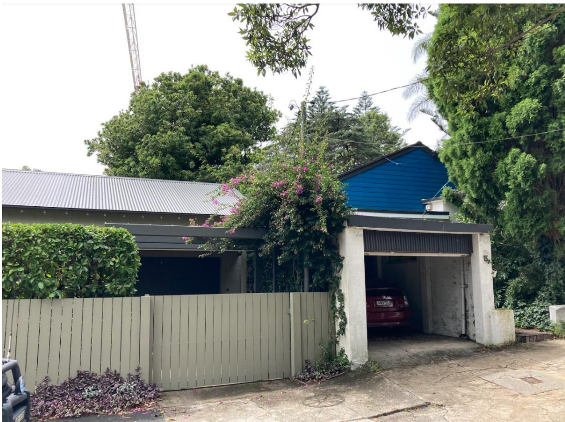
Figure 8: 14 (left) and 15 (right) Buller Street, viewed from end of Buller Street.
