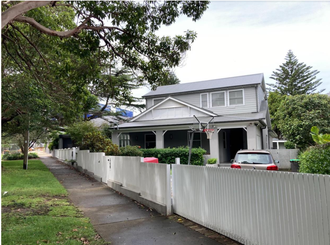
Figure 3: 13 Riddell Street, viewed from street frontage.
